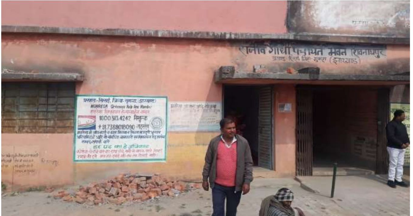
PANCHAYAT OFFICE GUMLA DISTRICT
