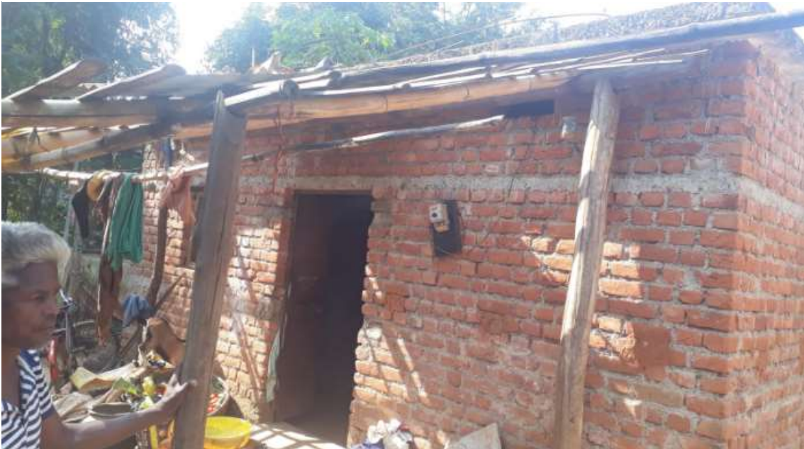
RURAL ELECTRIFICATION IN MALKANAGIRI DISTRICT
