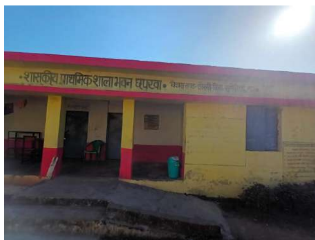
Photograph 9: Ramp for disabled students in Chhapparwa-Mungeli
