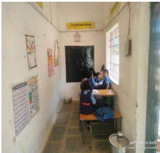
Photograph 17: Inappropriate classrooms in Rajnandgaon, Chhattisgarh
