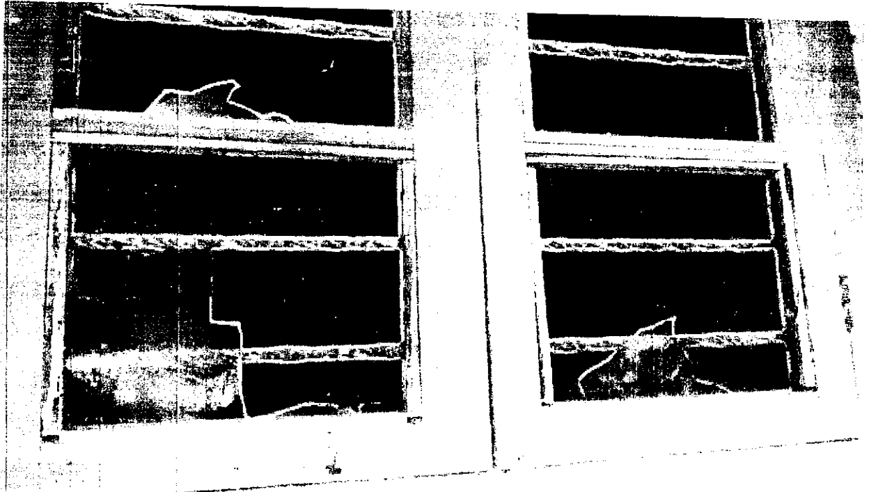
(Broken window glass, rusted grill)
