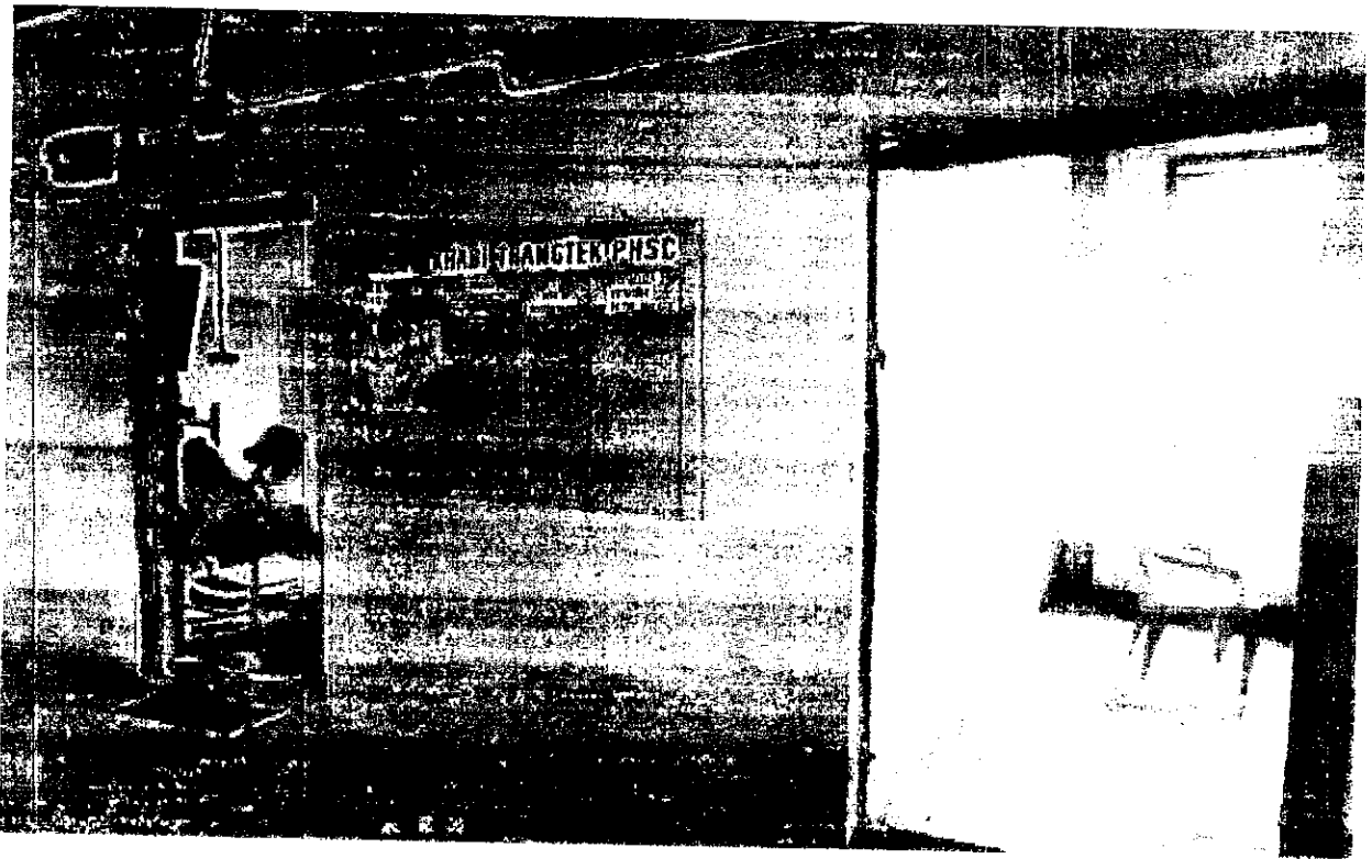
(An inside view of the PHSC taken from one of the broken windows)
